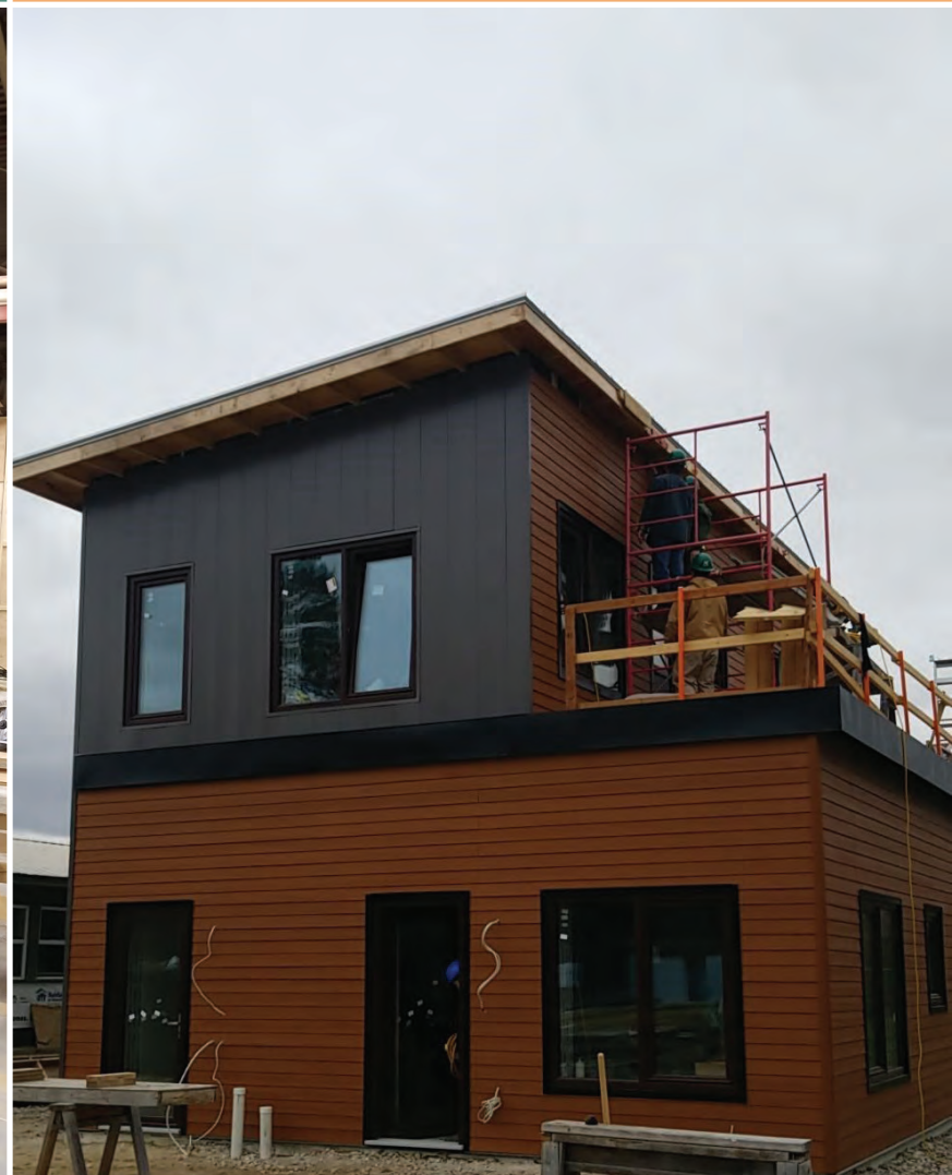
As part of the Carpentry Renovation Technician program Samuel and his fellow students helped to build this home in Perth, Ontario.
